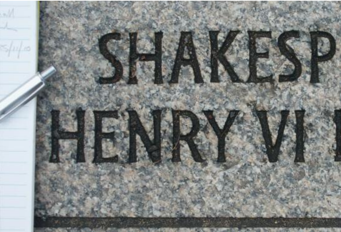
Two examples of sand-blasted lettering and design in London helped inform what could be achieved by sandblasting.
